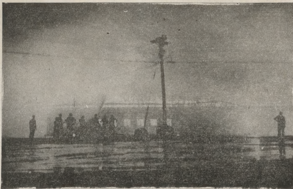
The flames were at their height when this picture was taken. The interior of the building that housed the bowling alleys has already been gutted and the roof is ablaze. See page 4.
